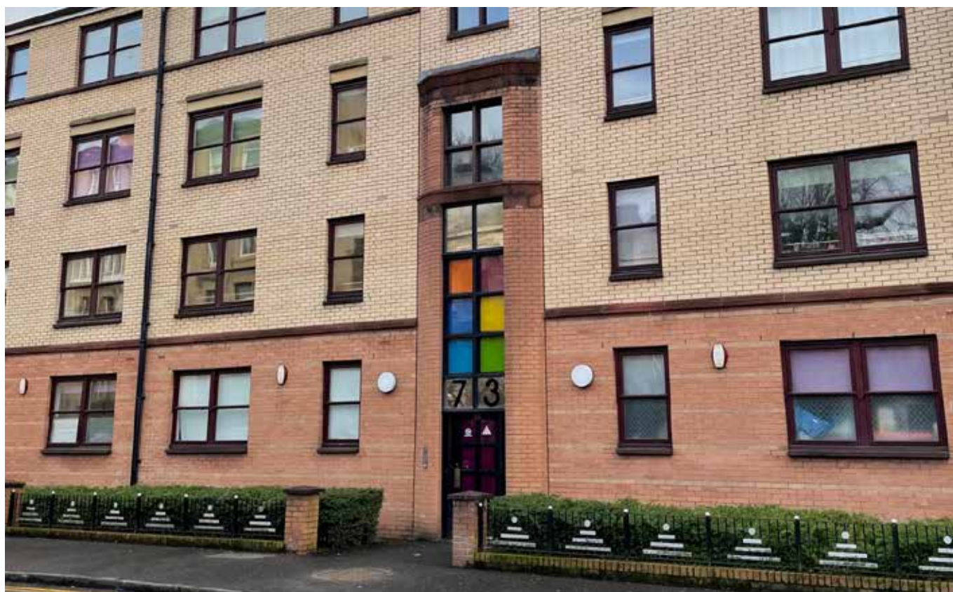
Above: A modern block of 12 flats in Glasgow was acquired.
